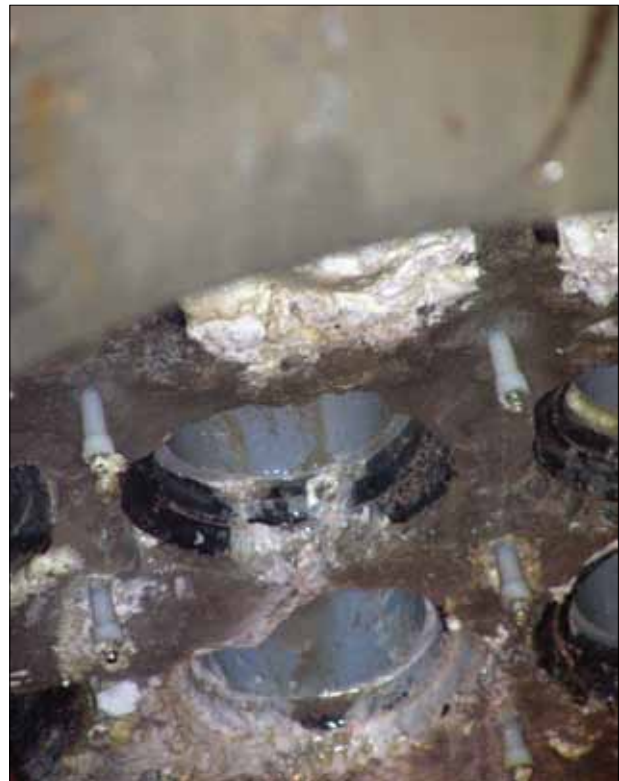
Figure 3 Close-up of the injection site.
