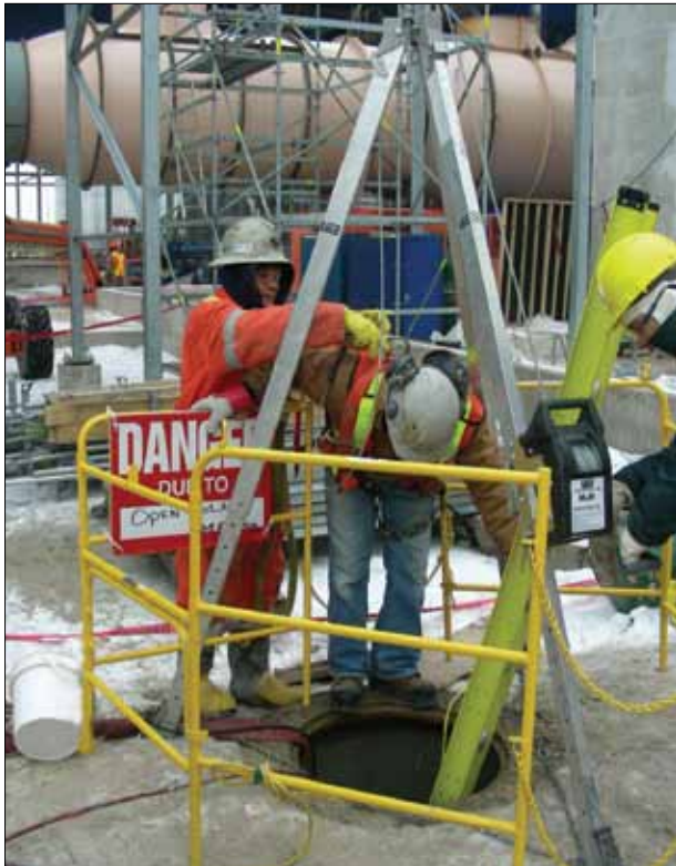
Figure 2 Preparing to enter the leaking manhole vaults during the injection process.
