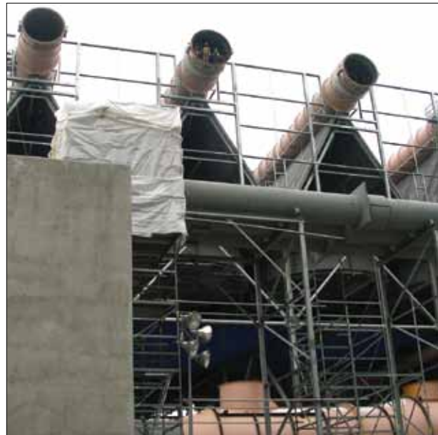
Figure 1 Goreway Station power plant under construction.
