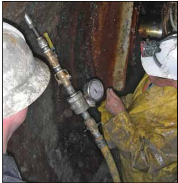
Figure 3 Injecting Azo-Grout™ 443 into packers in tunnel wall
