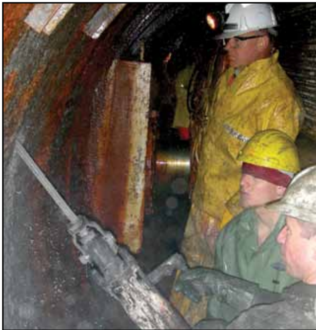
Figure 2 Drilling of injection holes prior to inserting packers
