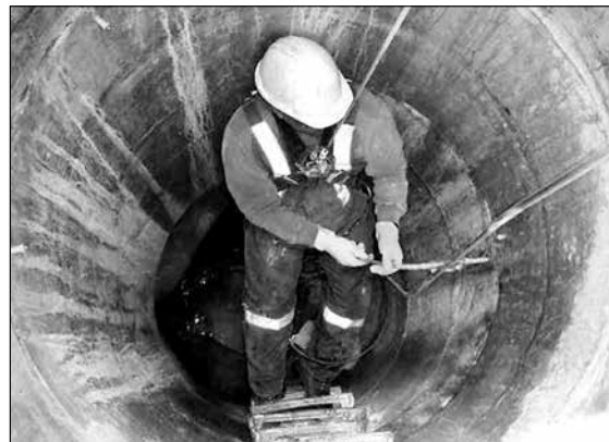
Manhole joint injection.
