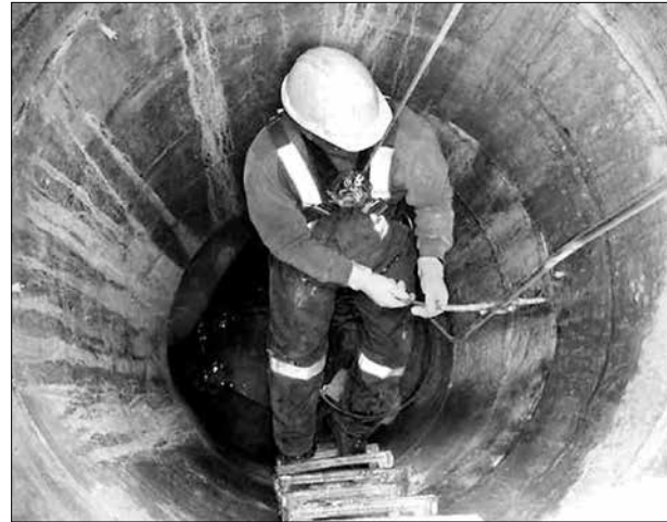
Manhole joint injection.
