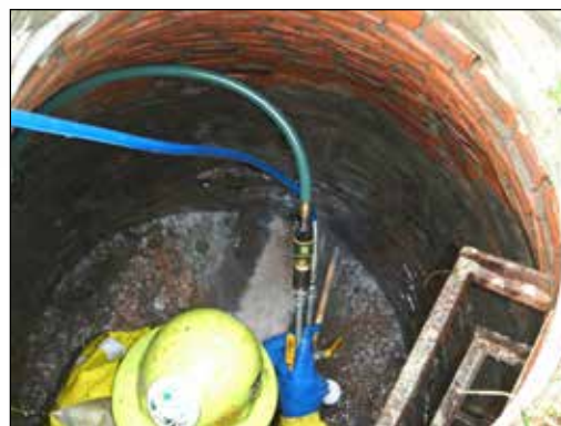
Azo-Grout™ being used in a manhole with a multi-ratio pump.
